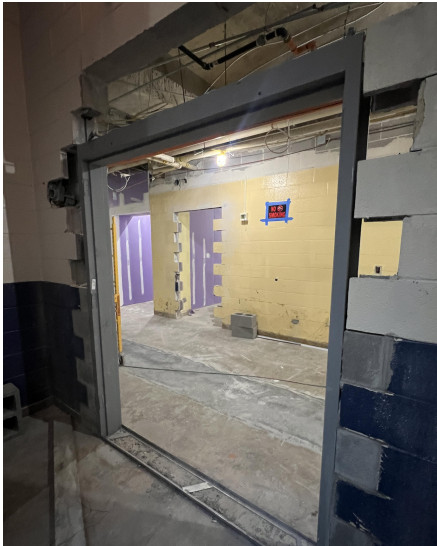
Setting door frames in the stairwell on level 1.
